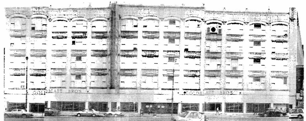
The five-story "addition" to the Goldblatt's store, at 1621-35 W. Chicago Ave., was built during 1925-28. It features large Chicago windows and a wealth of terra cotta details. (This photograph is a composite of four different photos, which accounts for the irregular nature of the roofline and storefronts.)
